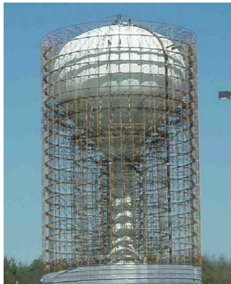
Tank scaffolding during project
