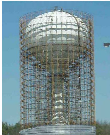
Tank scaffolding during project
