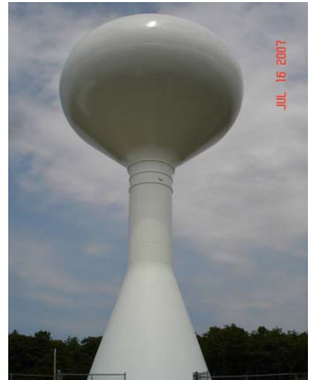
Tank after project completed
