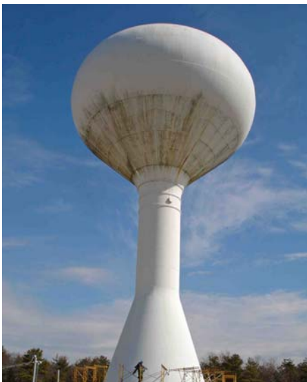
Condition of tank at start of project
