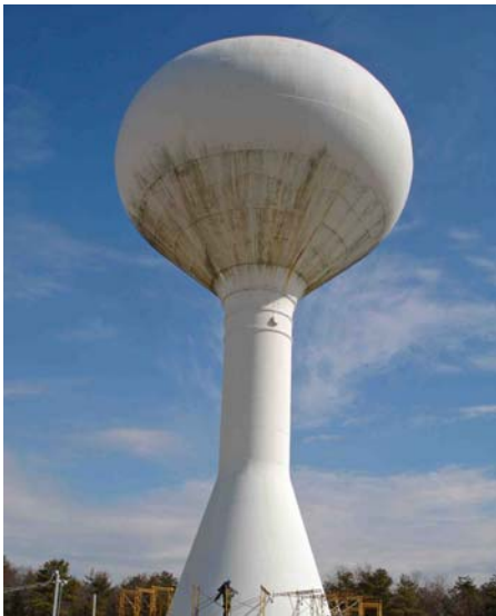
Condition of tank at start of project
