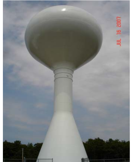
Tank after project completed
