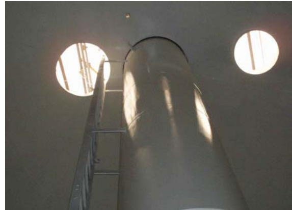
Roof and riser in tank’s exterior
