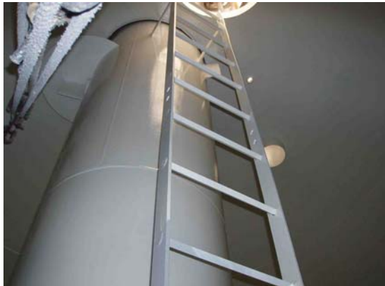
Roof and ladder in tank’s interior
