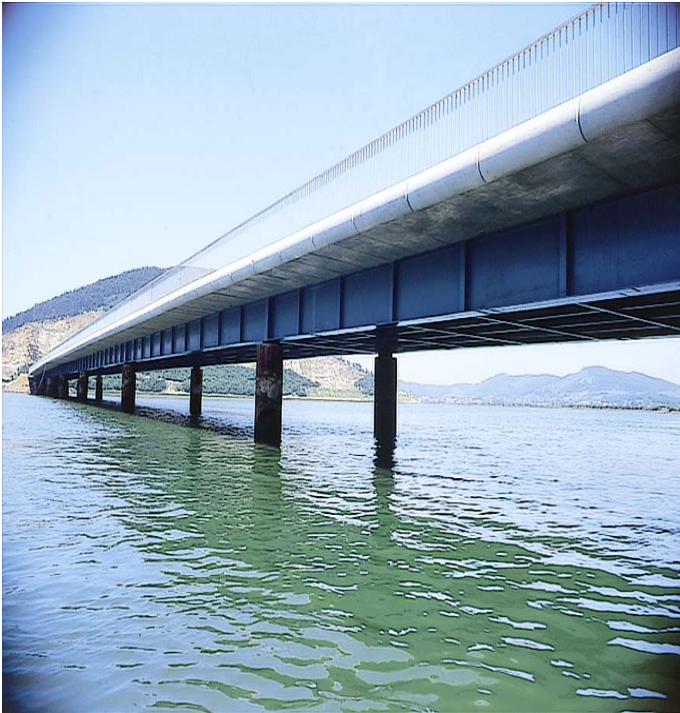
Estuary Entrance Bridge Santonia National Park, Spain
